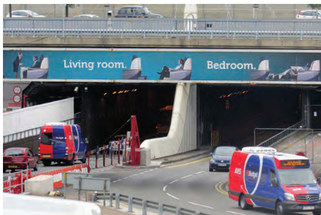
A view of the northern portals of the Heathrow Link Road Tunnel. There were road works taking place in the two outer tunnels when this picture was taken in 2014
